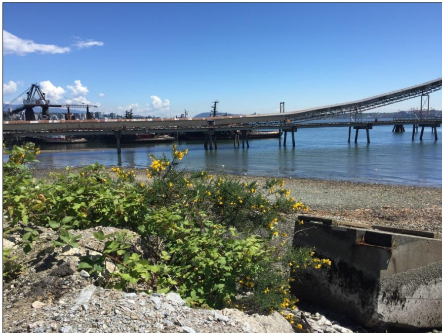
Photo 2 Rip-rap and vegetation looking south at Project site rail jetty modification area, west side
