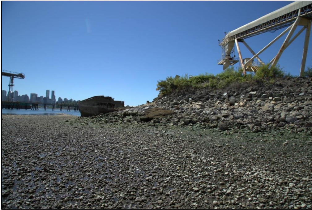
Photo 1: Rip-rap and foreshore looking west at Project Site rail jetty modification area, southeast side
