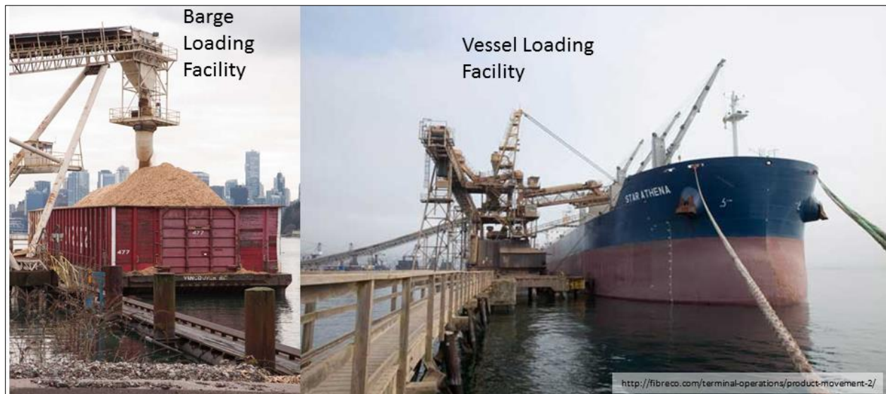
Photo 1 Barge Loading Facility and Vessel Loading Facility
