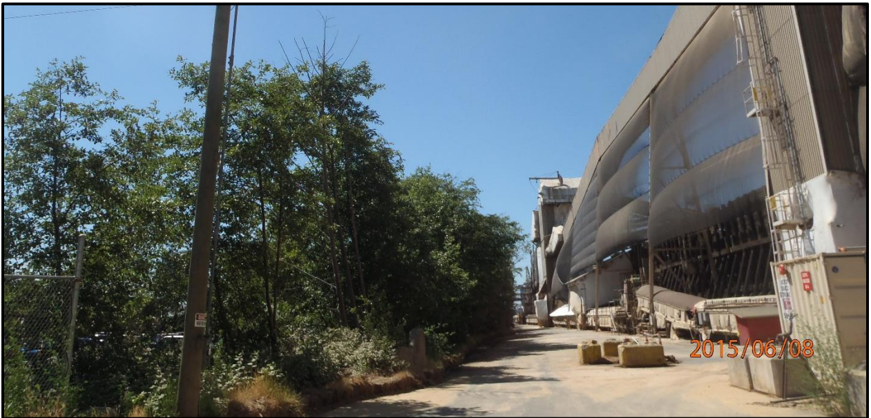
Photo 7 Riparian Area Along Eastern Side of the Site (looking south)
