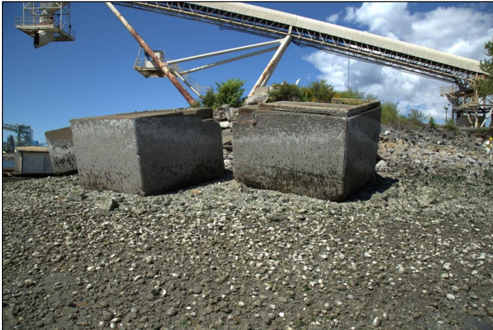
Photo 2: Cement blocks and rip-rap looking north at Project site jetty modification area, south side
